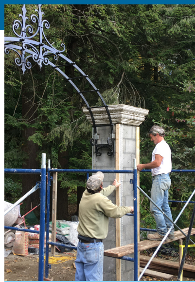
Studio Garden Arch restoration
